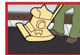
Step 1 - Lay approx. 50mm of crusher dust or paving sand. Screed the base off to the required level. Dampen base and compact by hand or with a vibrating plate compactor machine.
