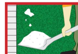
Step 4 - Cover entire area of Prograss using a ballast layer of clean sand and/or granulated rubber allowing extra around the edges and in the corners.
